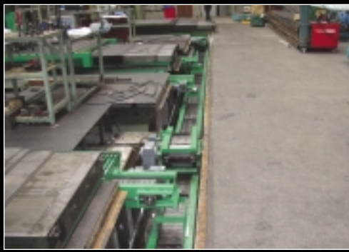
Full Factory Installation of 17 Conveyors
